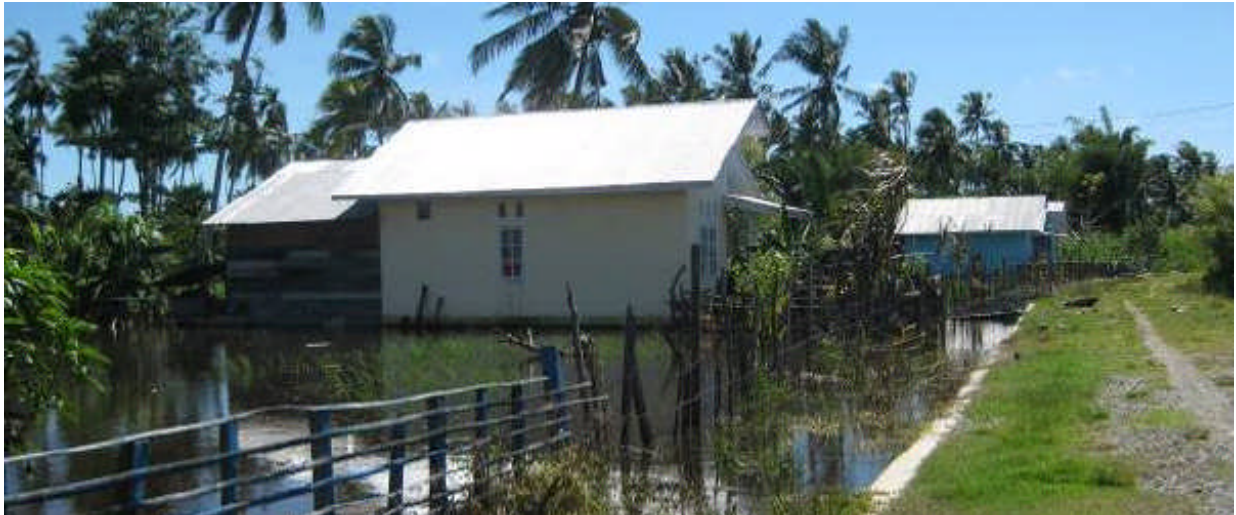
Figure 2: Flooded houses in Indonesia at the time of the assessment
